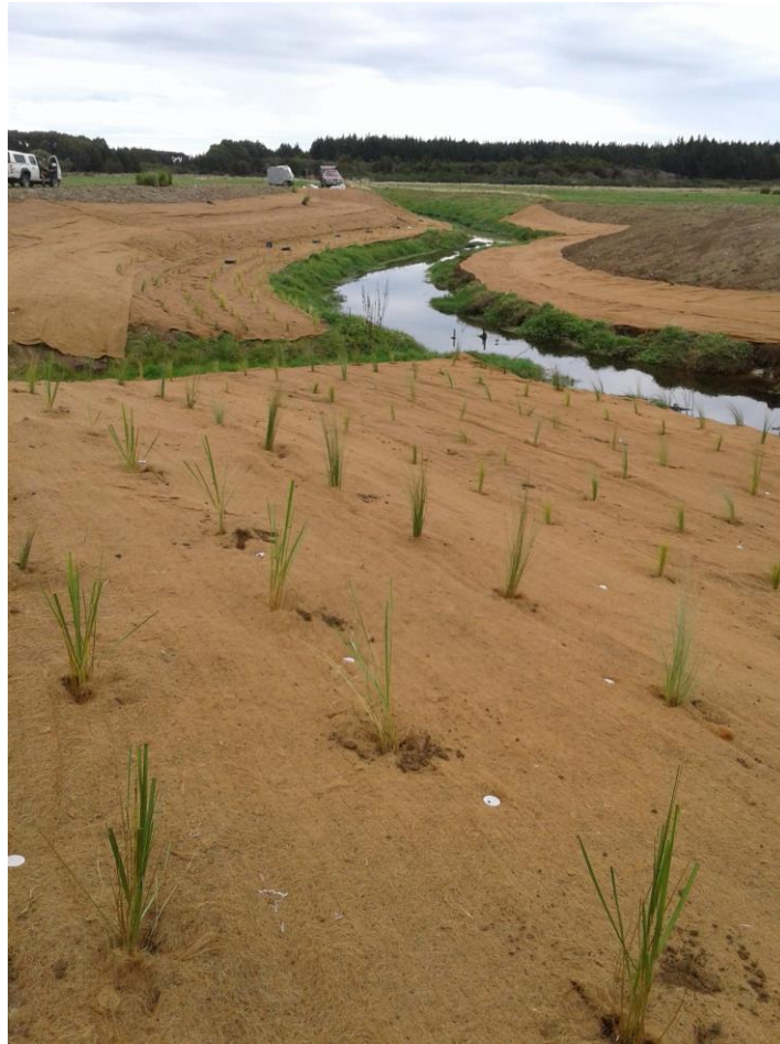
Figure 5. The Site 2 rehabilitation reach showing recent plantings and two-stage channel design, photograph taken in 2018 from bank-full looking downstream.
