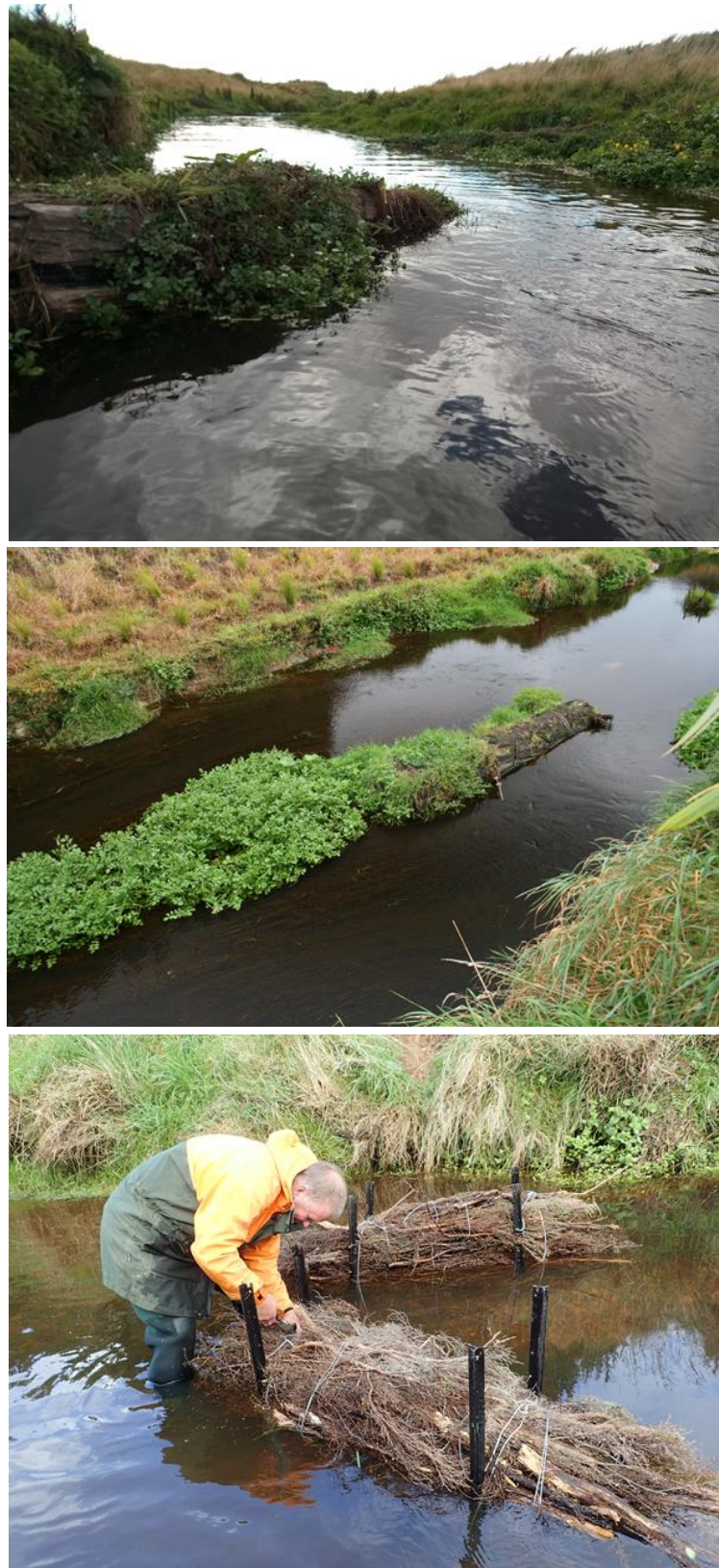
Figure 3. Waituna Creek showing examples of the logs (top and middle) and manuka bundles (bottom) installed within the rehabilitation trial reaches to improve fish habitat (figures reproduced from Holmes 2019a).
