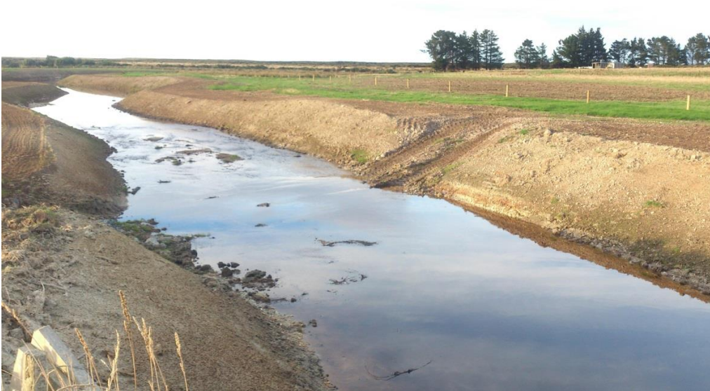
Figure 1. Bank re-shaping in a reach of the lower Waituna Creek (March 2014)
