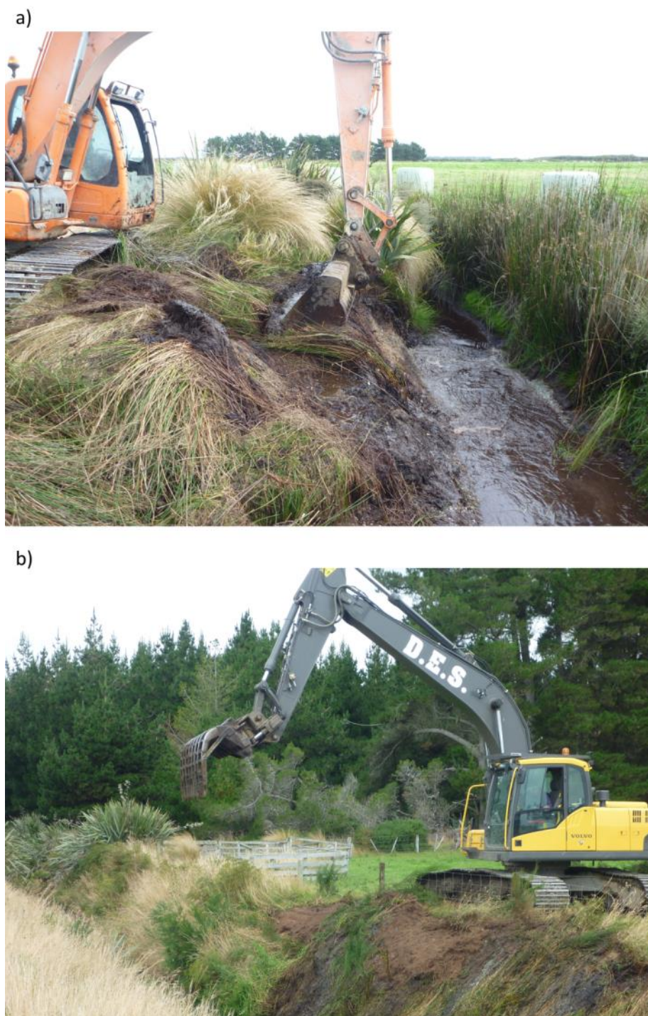
Figure 5.2 Photograph of the two attachments used while excavating the study sites. a) Depicts a standard bucket similar to that used to excavate silt and plant material from Russell Outlet and Hautapu. b) Depicts a weed rake similar to that used to excavated plant material from Affco.
