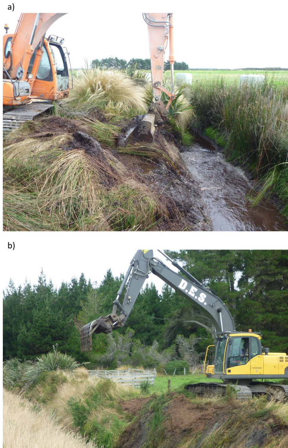
Figure 3.2 Photograph of the two attachments used while excavating the study sites. a) Depicts the perforated bucket used to excavate silt and plant material from Armstrong, Carran 1 and Moffat 1 during experimental excavation in 2011. b) Depicts the weed rake used to excavate plant material from the remaining sites in 2012.
