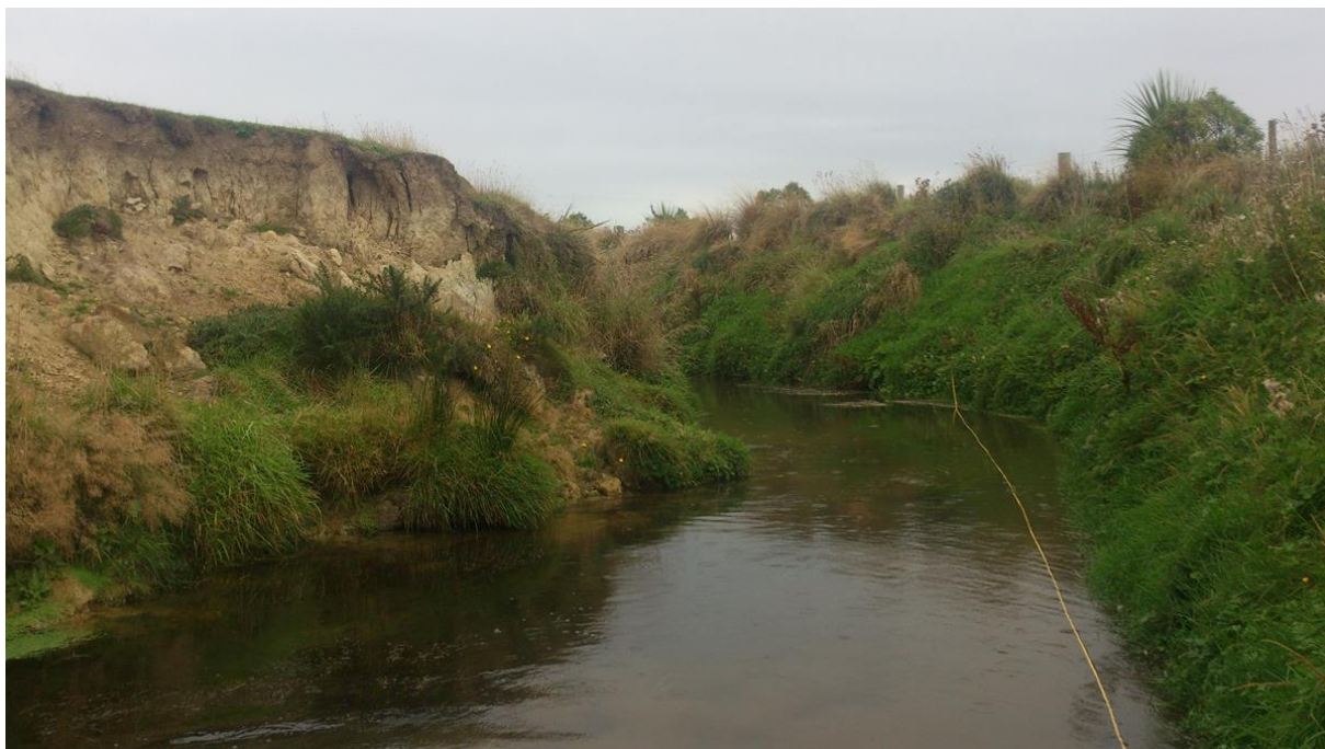
Figure 12. Waituna Creek (mid catchment) looking downstream. On the true left, mass failure of the bank (bank slumping) can be seen on the inside bend of the stream that is accessible to stock ( i.e. no stock exclusion fencing). The riparian area of the inside bend (right) has been fenced from stock for at least 5 years.
