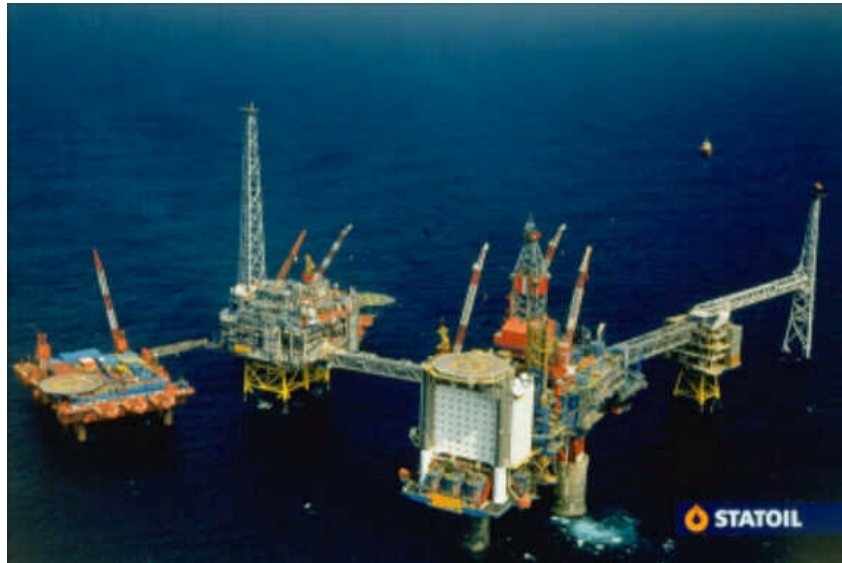
Sleipner natural gas field, site of the first commercial scale CO 2 storage in an aquifer (Statoil)
