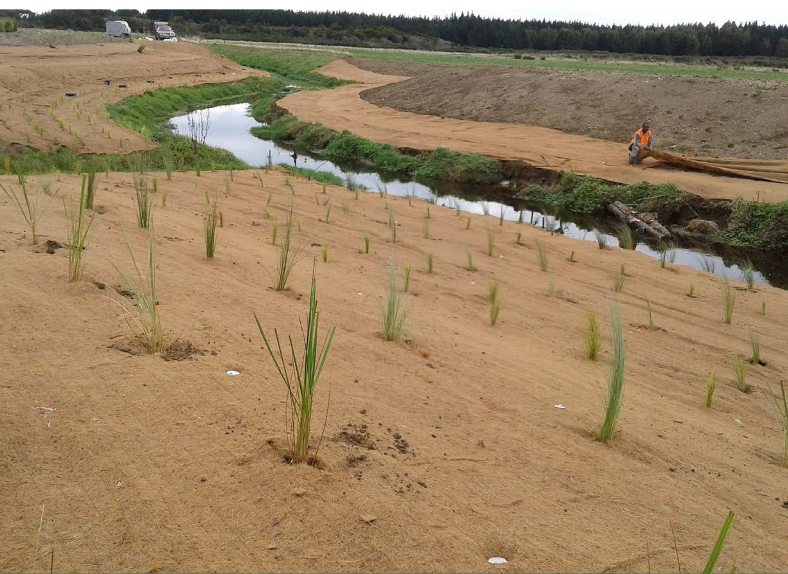
Early plantings along Waituna Creek after the re-shaping of the banks.
