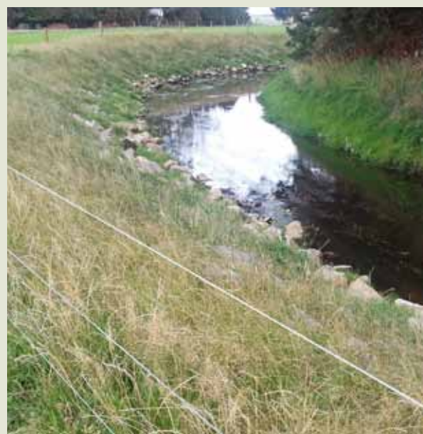
After the completion of reconstruction work.
