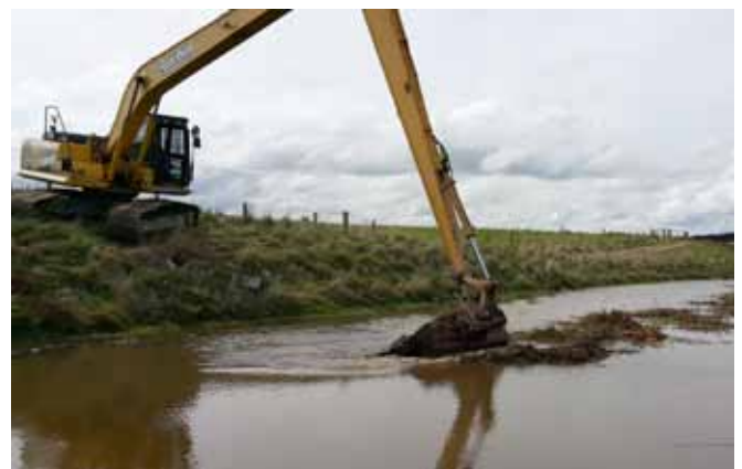
Eleocharis is transplanted to a constructed wetland trial area.
