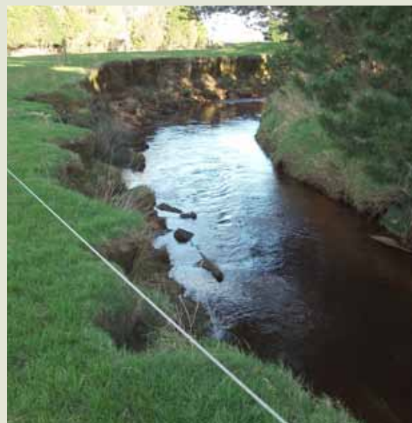
Before work started on bank reconstruction along the Waituna Creek.
