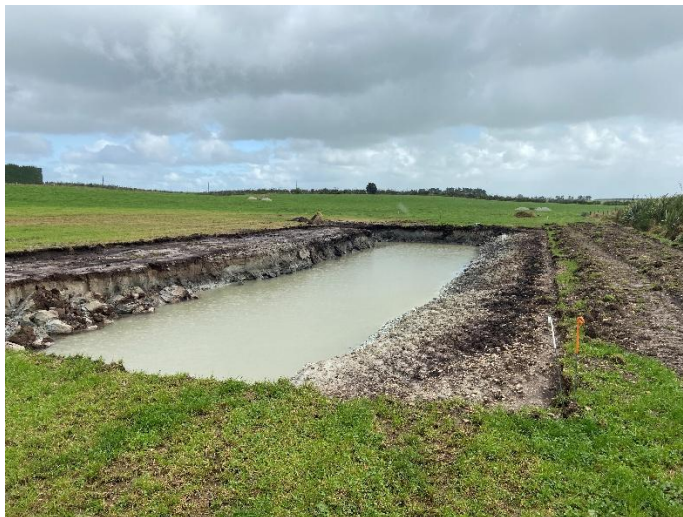
Sediment trap under construction March 2023
