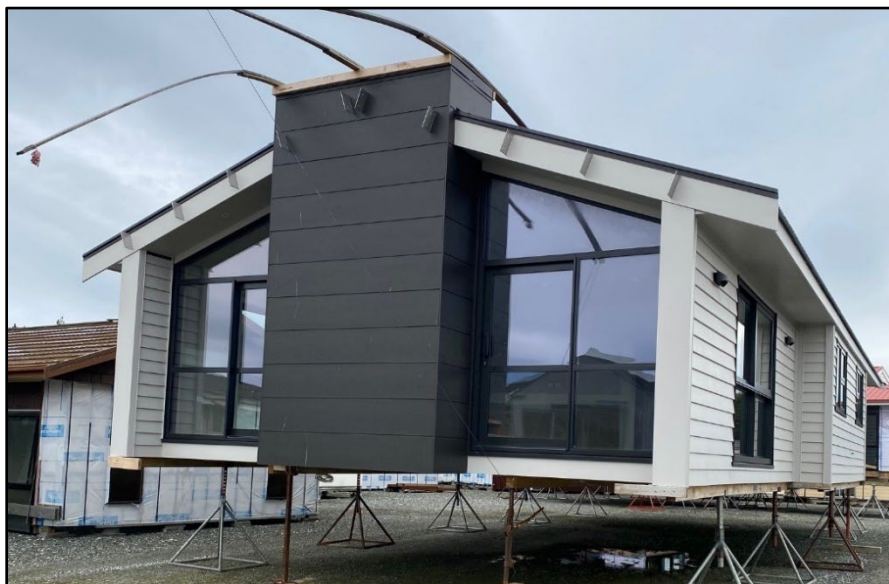
Completed Cultural Centre ready to be moved onto the Mahinga Kai Pa site in FY24/25.
