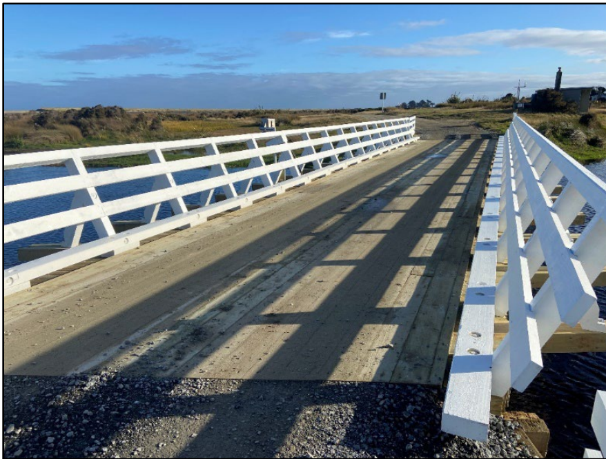
New bridge completed – March 2024
