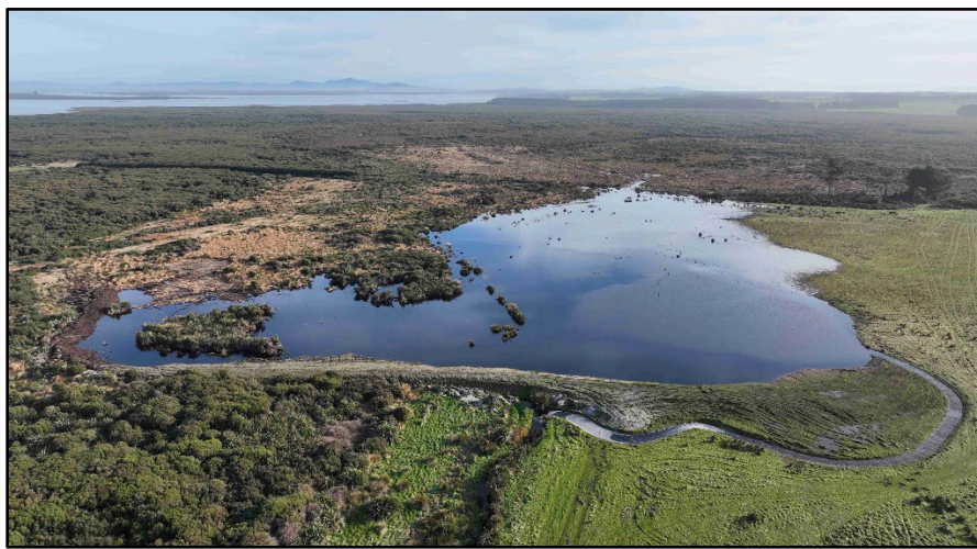
Third wetland, completed on the western side of the Mahinga Kai Pa.
