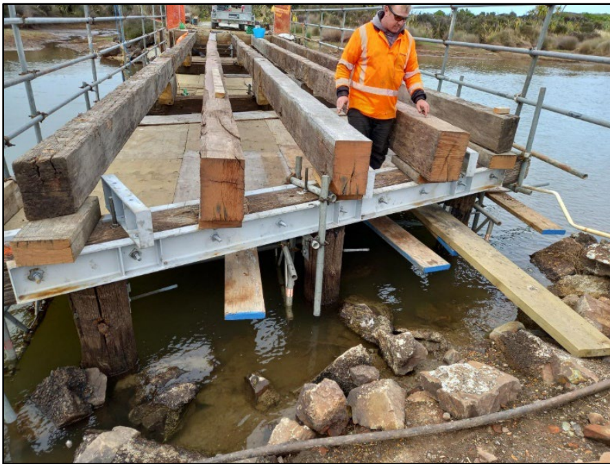
New bridge base being installed – February 2024
